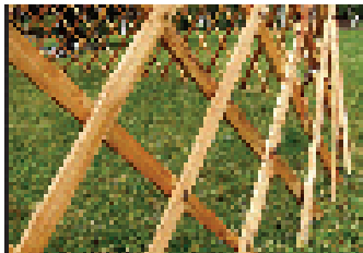
• It is possible to unfurl and furl this like cervical vertebrae. What is this? ( Lattice wall of ger )
