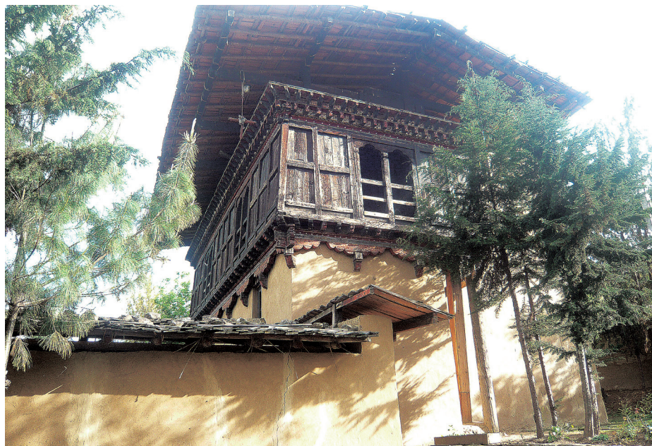
Folk Heritage Museum of Bhutan (Photo by the Folk Heritage Museum, Bhutan)
